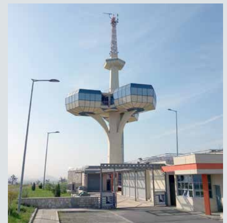
The Montenegro control and monitoring center (GKMC) is equipped with a Rohde & Schwarz monitoring system.
